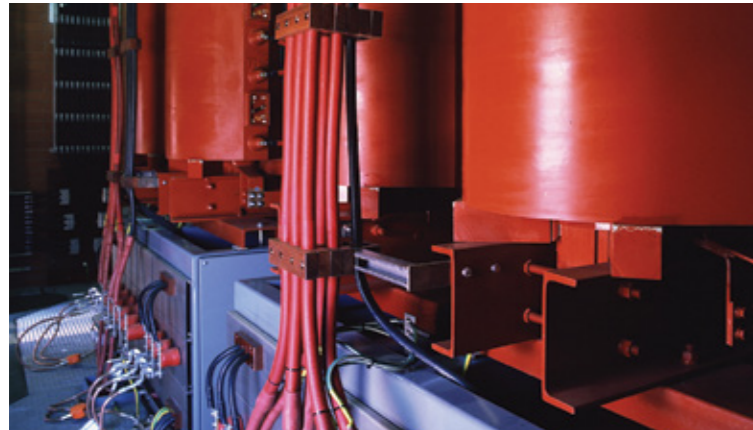
2.5MVA power transformer installation
